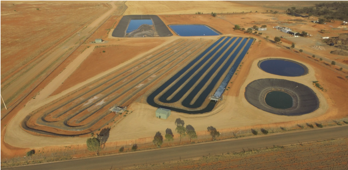
District Council of Peterborough’s CWMS scheme showing the high-rate algal ponds. The CWMS scheme cost $21 million.
