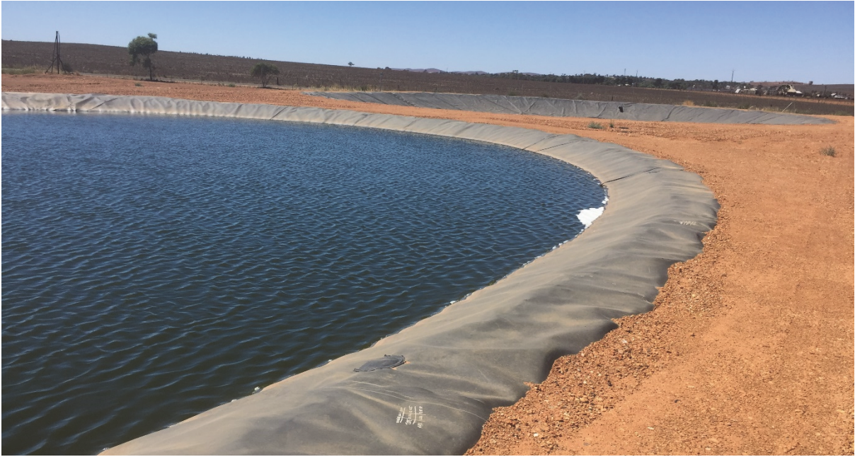
District Council of Peterborough's wastewater treatment plant anaerobic lagoon.
