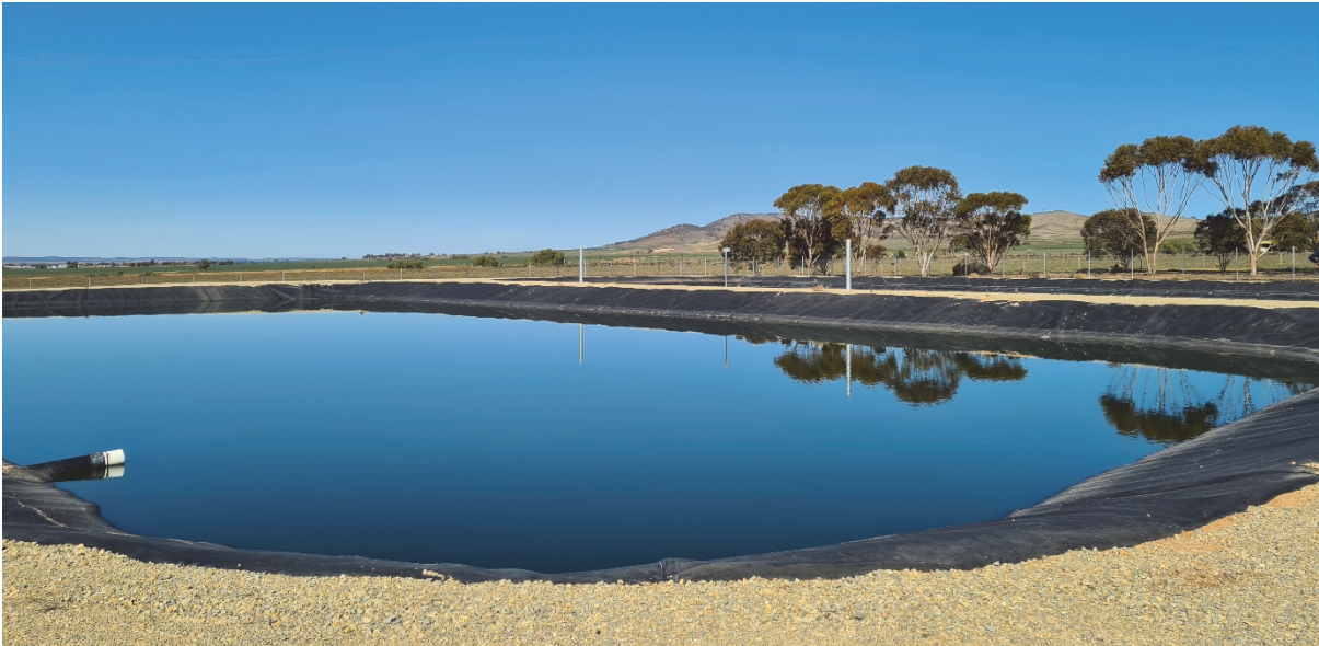
District Council of Orroroo’s wastewater treatment plant lagoon. The CWMS scheme cost $2.12 million.
