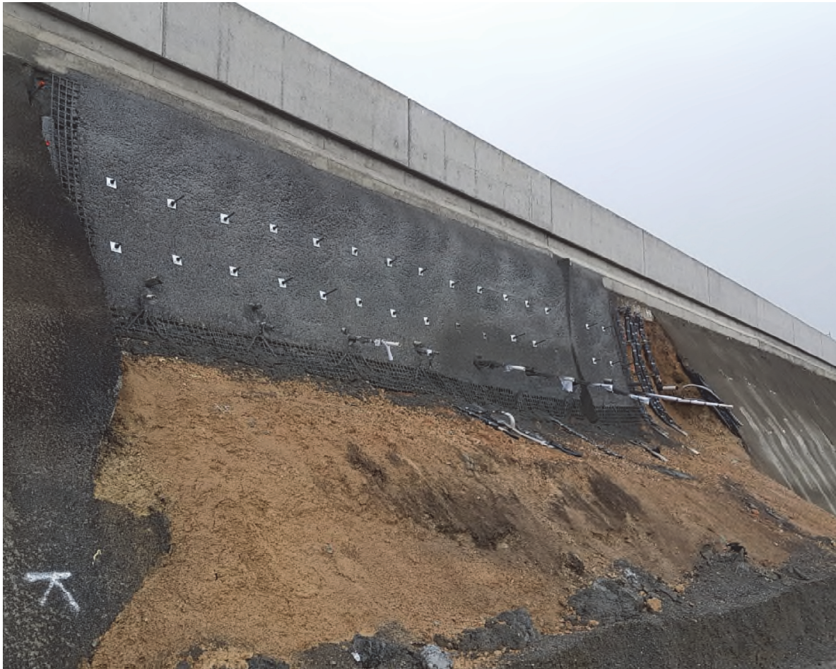
Figure 4.7: Repair works to RW 1102
