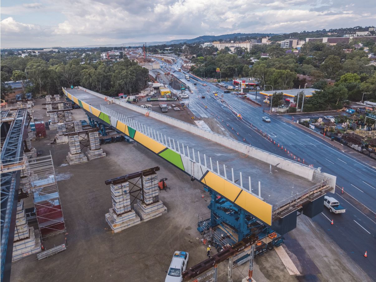
Figure 2.8: DUP bridge on self-propelled modular transporters
