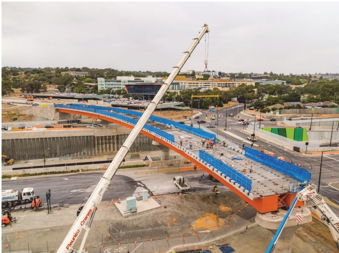
Figure 2.4: Installation of elevated rail bridge span
