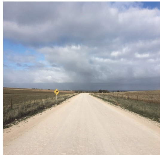
Resheeted unsealed road
